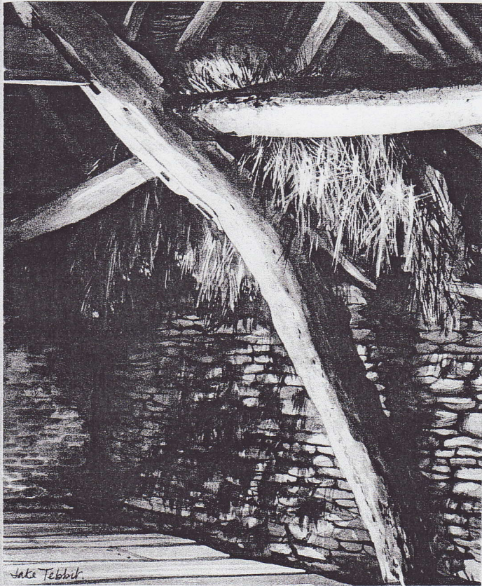
One of the original cruck beams, installed when the longhouse was built.
