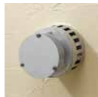
Balanced Flue (No chimney required) BF
